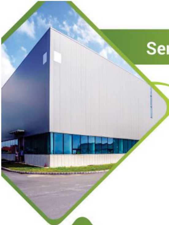
Elevation Glazing and Aluminum Composite Paneling
