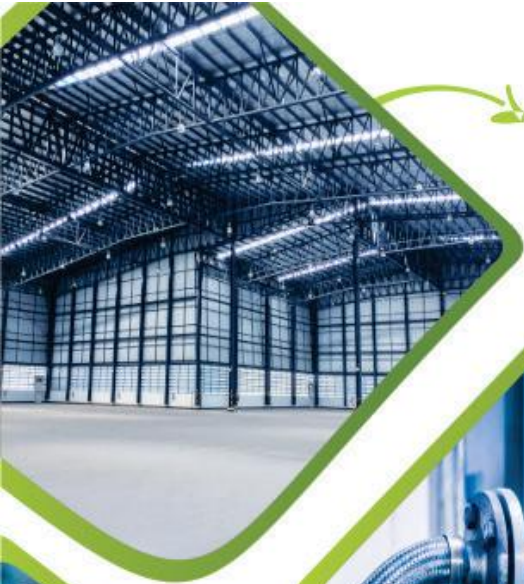
Roof Structures and Sheeting
